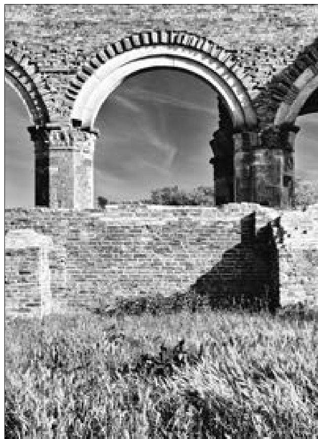
▲ Arches in Arcade in Romanesque style; Photo: L. Lazić
